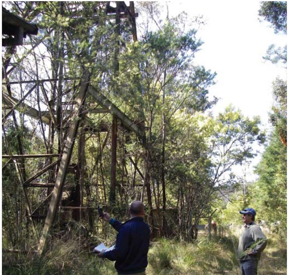
An historic head frame at Bielsdown, which was used for a shaft that was previously sunk to a depth of 165 metres.
